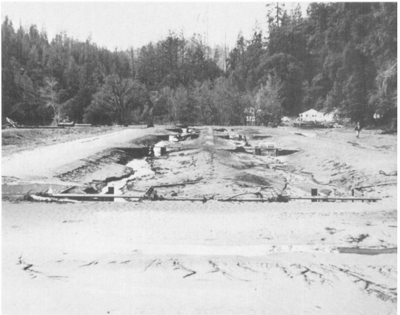
FIGURE 47. Cedar Creek Hatchery ponds after inundation by flood, December 1955. Department of Fish and Game photograph, December 26, 1955.
