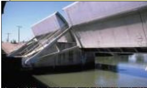
Moveable gates to the Delta Cross Channel. Open, the gates allowed tidal flows of about 9,000 cubic feet per second (cfs) and net flows of about 4,000 cfs to pass through the channel, according to fall 2000 hydrodynamic monitoring.
