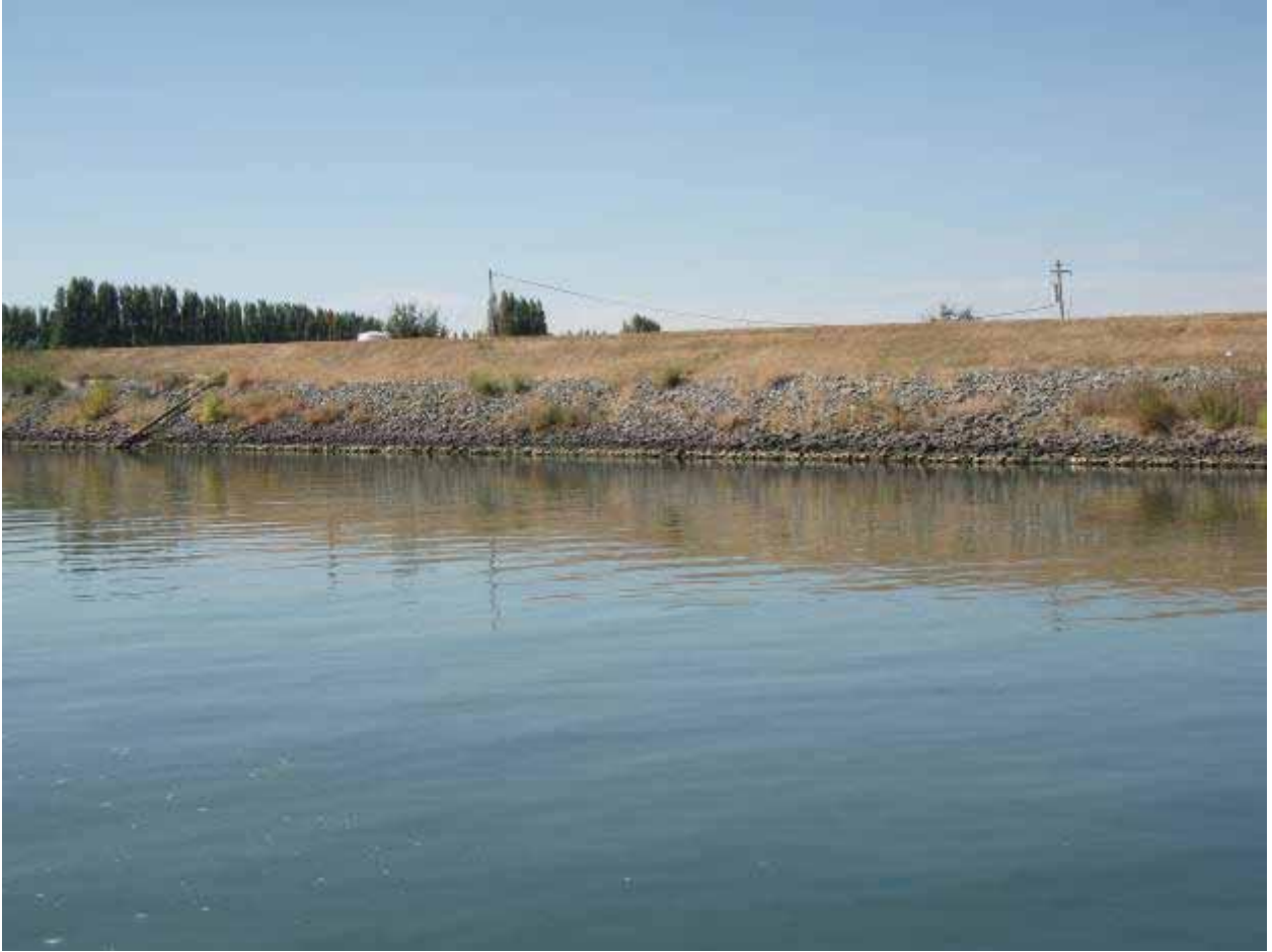
Figure C-1 Sacramento River south of Courtland, showing repair of erosion using rip-rap
