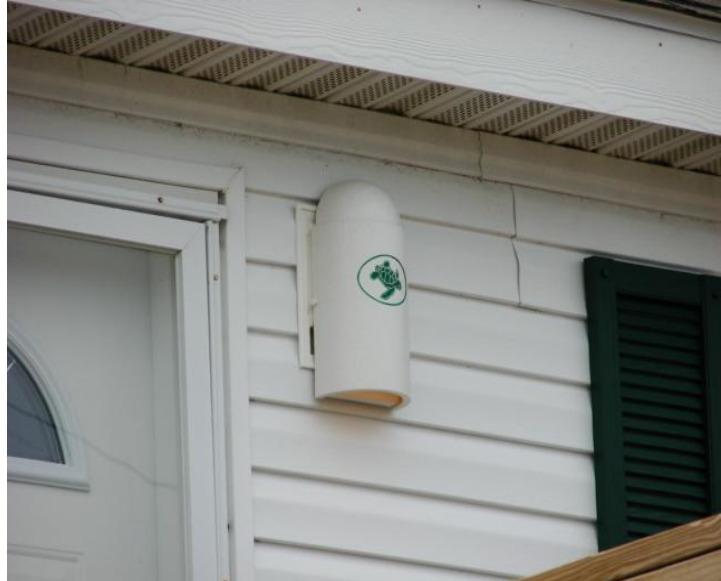
Figure 2. Onslow Beach housing unit showing canister lighting.
