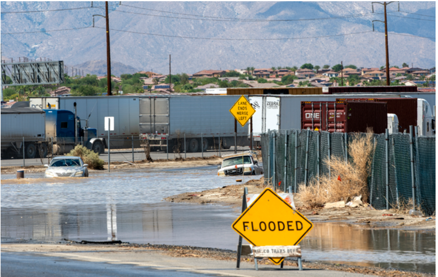
Vehicles became inundated with water while trying to use a road which was flooded by Tropical Storm Hilary to bypass traffic on Interstate 10 near Thousand Palms, CA on August 21, 2023.
