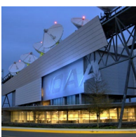
NOAA's Satellite Operations Facility in Suitland, Maryland. Photo credit: NOAA Photo Library, NOAA Satellites .
